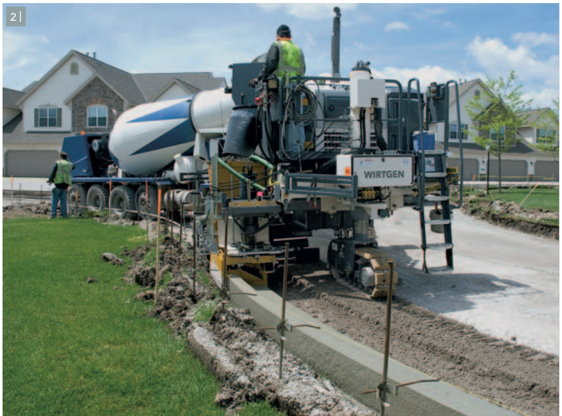
2 | No problem: highly accurate paving of radii with the SP 15/SP 15i.
