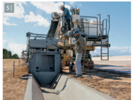
3 | Paving pedestrian and bicycle paths at widths of up to 1.8 m using a mould offering modular extension.
