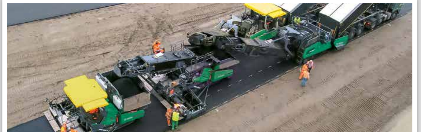
FEEDING PAVERS IN AN INLINE PAVE TRAIN
